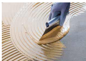
Picture 1. Trowel spread
